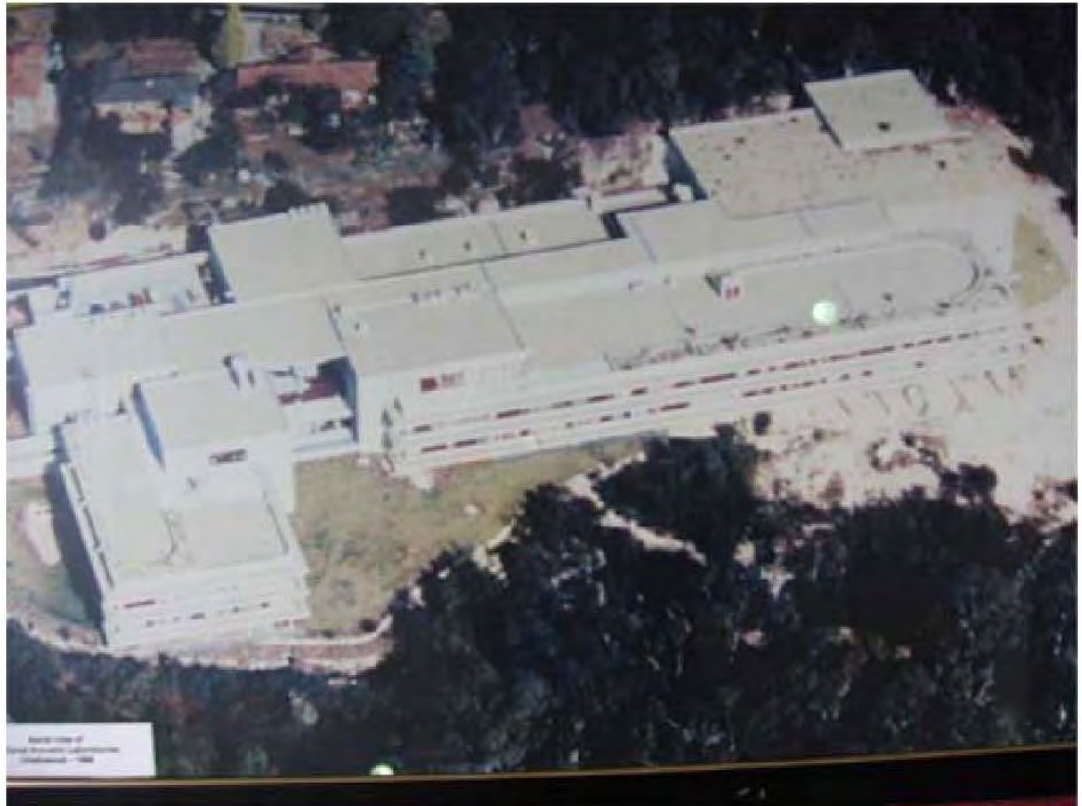
Plate 4: Aerial photograph of the site near completion
